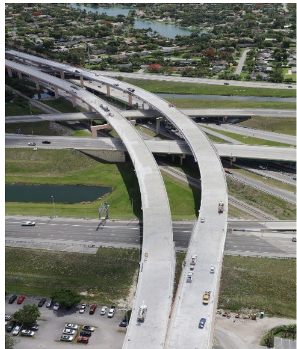
SR 874 Northbound/Southbound Connector Bridges to SR 874
